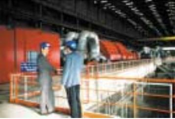
As operational demands continue to increase, the one area that cannot be compromised is safety. Safety will always be a paramount concern for turbogenerator operations, due to potential explosions caused by air mixing with hydrogen. The ABB hydrogen analysis system eases the stress of working in hazardous environments by providing continuous, reliable monitoring of hydrogen purity without fail.
